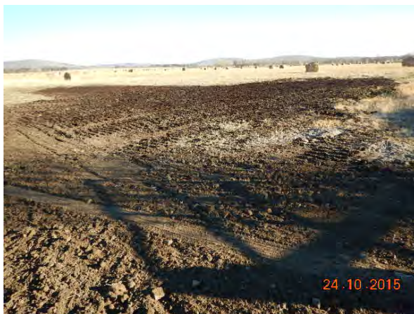
Photo 5. Work completed to re-establish grade, install topsoil, track pack and seed to repair livestock damage at KP 9.050 (October 24, 2015).
