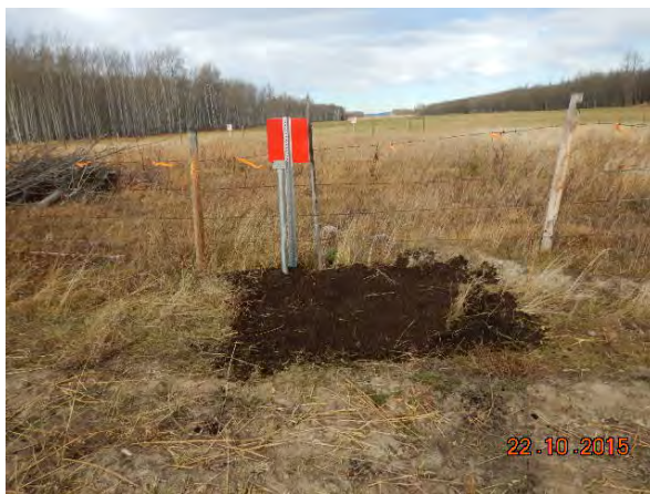
Photo 9. Added topsoil, packed and seeded minor subsidence just west of the T-North 2012 ROW as per the landowners request (October 22, 2015)..
