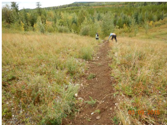
Photo 20a. Same general view as Photo 20 showing good vegetation and coverage on the slope and repairs to the diversion berm ( September 3, 2015 ).
