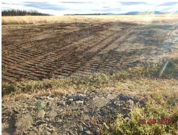
Photo 3. Repairs underway at KP 4.060 to correct drainage issues caused by recent clean-up on an adjacent line and landowner water management practices (October 23, 2015).
