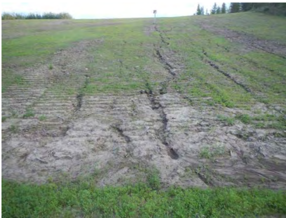
Photo 17. View south of the right-of-way and rill erosion on the south approach slope to Portage Creek at KP 17.958 (August 28, 2013).
