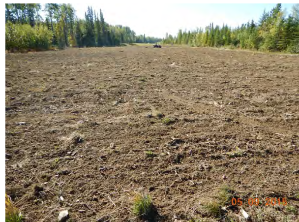
Photo 12. Looking south from KP 18.550 at the disking completed by the landowner and seeding completed by the contractor to address erosion and the lack of vegetation as a results of seeding not being completed by the landowner as committed (September 5, 2015)
