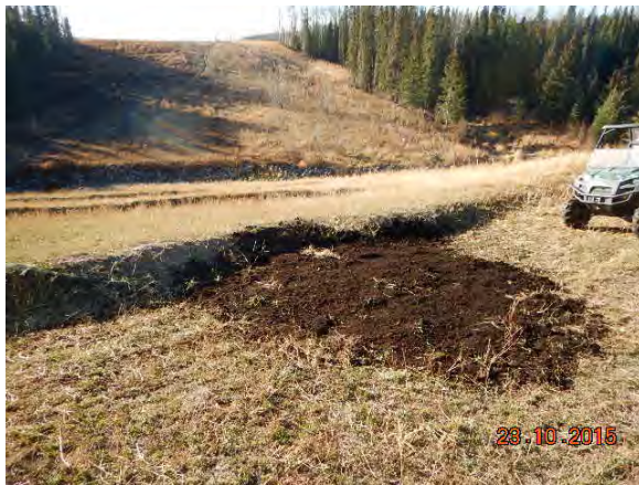
Photo 7. Topsoil placed for packing and seeding to repair the surface breaker and compaction / water ponding caused by livestock overuse on the north slope of Brenot Creek at KP 12.710 (October 23, 2015).
