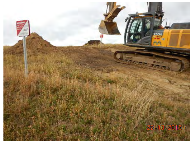
Photo 10. Topsoil was stripped and the erosion gullies on the slope at KP 17.920 were filled with shale and compacted to prevent further erosion (October 22, 2015).
