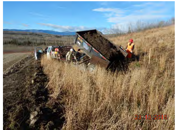
Photo 2. Ground crew in the process of filling the minor bellhole subsidence at KP 2.570 prior to packing, seeding and applying fertilizer (October 23, 2015).
