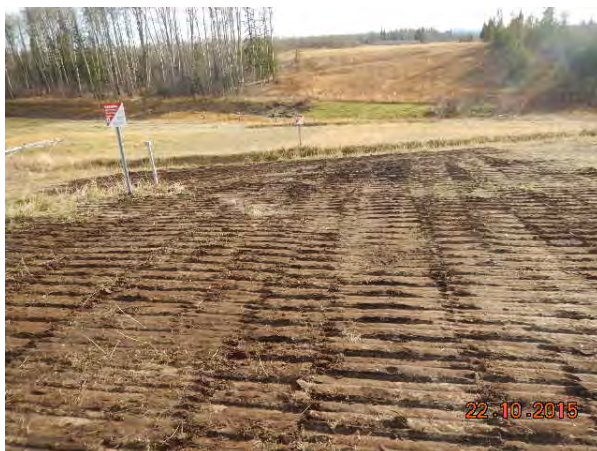
Photo 11. Topsoil was then replaced and seeding and track packing was completed at KP 17.920 (October 22, 2015).
