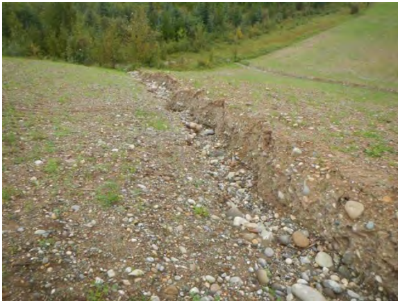
Photo 20. View northwest across the right-of-way and gully erosion along a diversion berm ( August 27, 2013 ).
