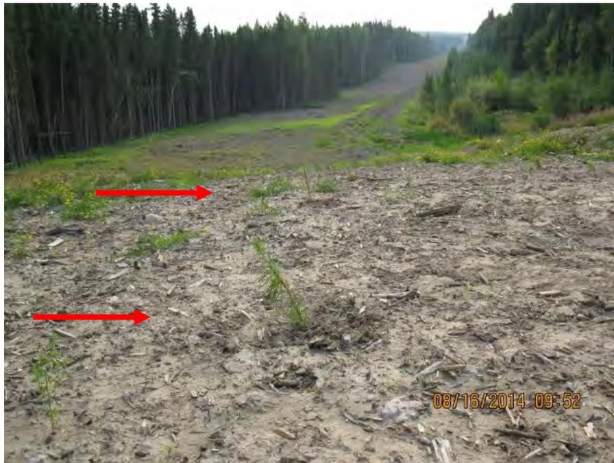
Plate 3: Example of conifer seedling planting on a pipeline ROW. The upland area has sufficient drainage and suitable soils for seedling establishment and growth. Photo source: CH2M HILL.
