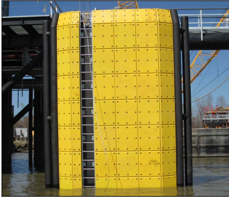
FIGURE 3-2: PHOTOGRAPH OF EXAMPLE FENDER PANEL WITH 100 MT CAPACITY FENDER POSTS
