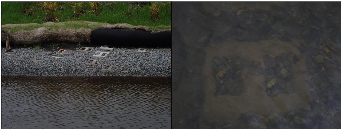
Figure 3: Stewart Creek at Transmountain Pipeline Crossing on December 12, 2018. The stream bed is completely lined with concrete blocks.
